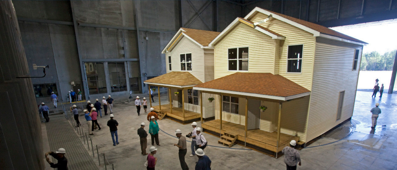
Home built to conventional Midwest construction standards (L) and home built to IBHS FORTIFIED for Safer Living ® standards (R) in IBHS Research Center test chamber.
